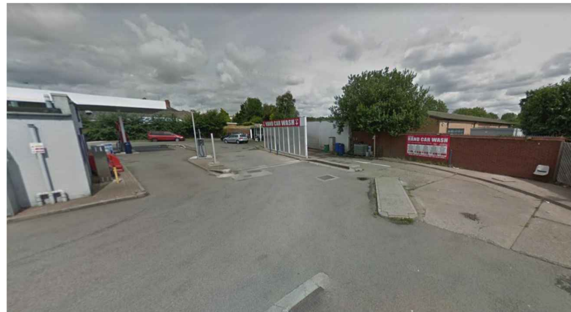
Image E - Petrol Station Service Yard
